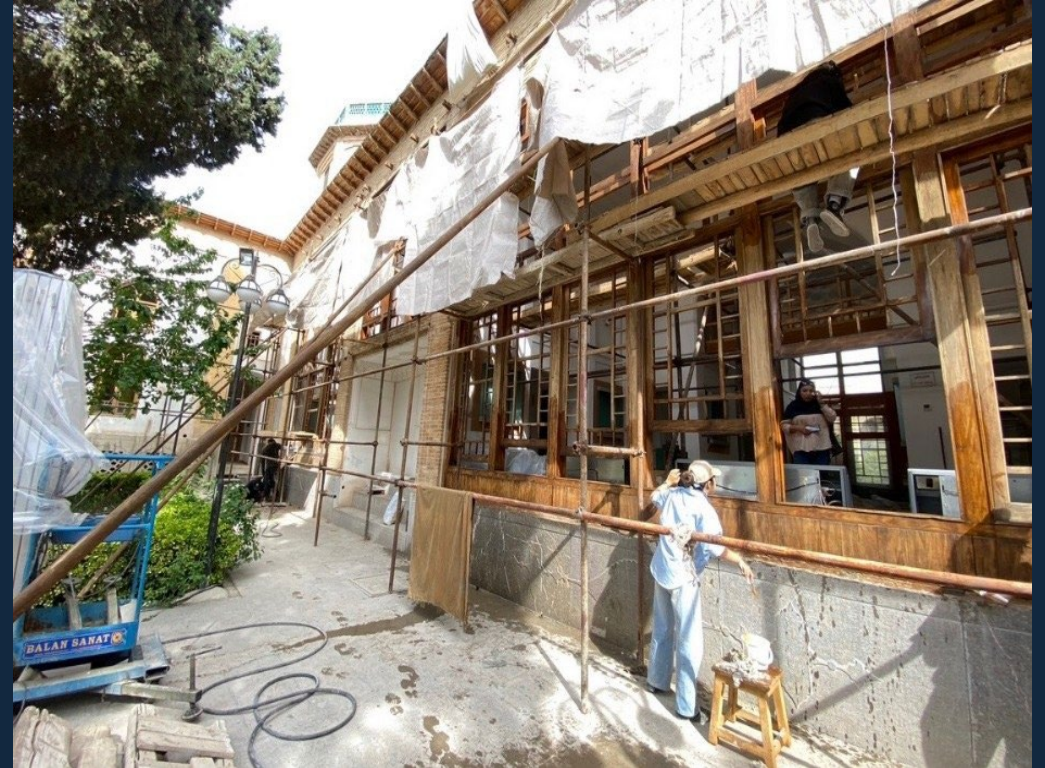
Temporary sheeting to windows and doors after the Ramadan war
