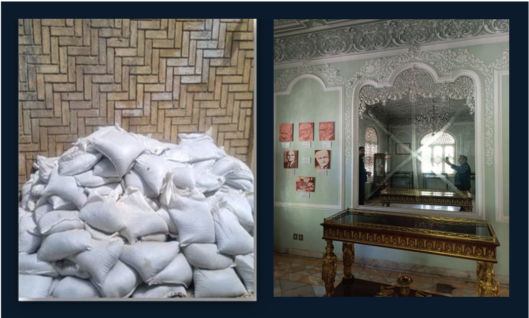
Sandbag walls staged to absorb blast energy
