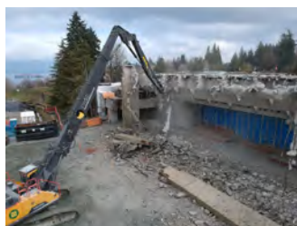
Volvo EC480E High Reach Demolition
