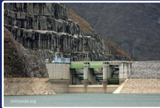
Chixoy Dam · Photos: James Rodríguez / mimundo.org
